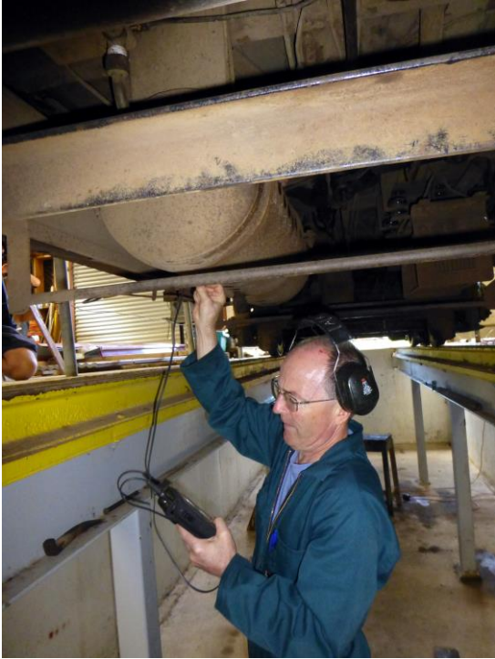
Above: Alan Caldwell, of Engineering Quality Testing Ltd., carries out ultrasonic thickness measurement on the air tank of tram 159 on 28 th January.
