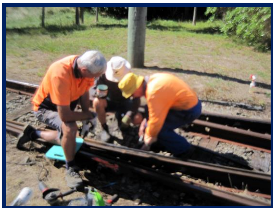
Above: Track maintenance at the loop, 2 nd March 2019 – replacing fishplate bolts.
