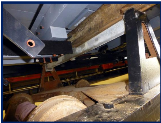
Above: A view under tram 17 of the modified Sammy truck mounting arrangement that allowed the tram to traverse curves.
